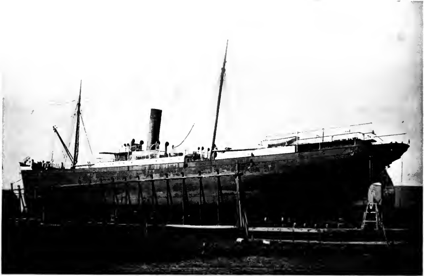
The 3,500-ton Crandall dock at the Alameda plant of the Union Iron Works Company.
